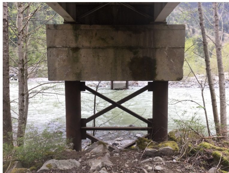
Left bank pier left face
