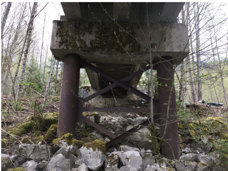
Left bank pier right face
