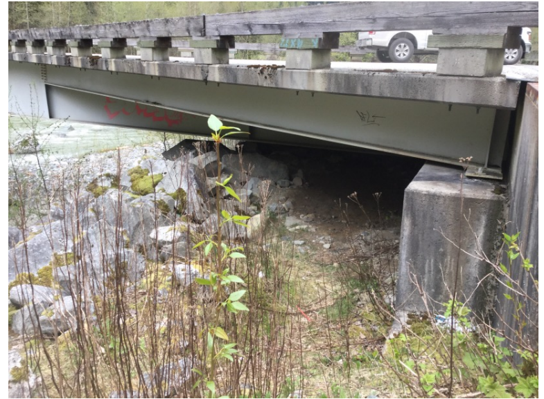
Upstream right bank flared girder
