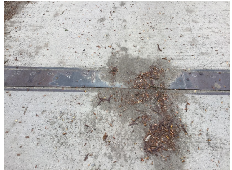
Left span to center span deck joint
