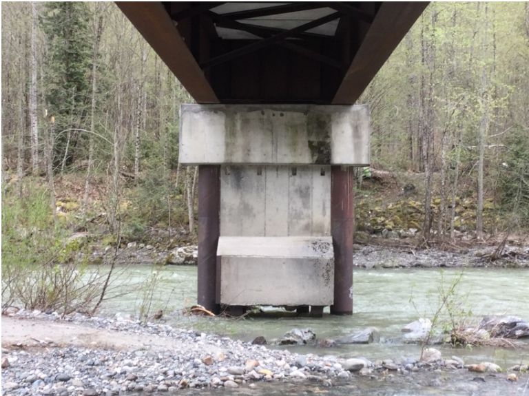
Right pier right face
