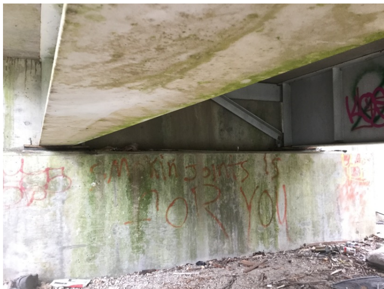
Left Bank Abutment when facing downstream
